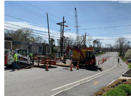
In-road sewer excavation has concluded for the season
